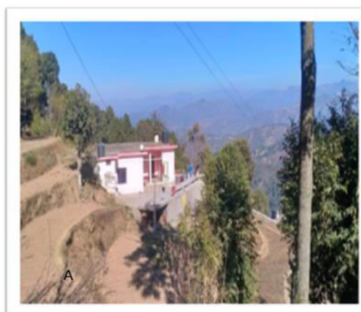
Figure 5A. Pucca house with retaining wall made of local stone.
