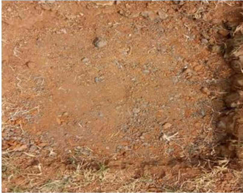
Fig. 3.3: clayey soil replaced with sand layer
